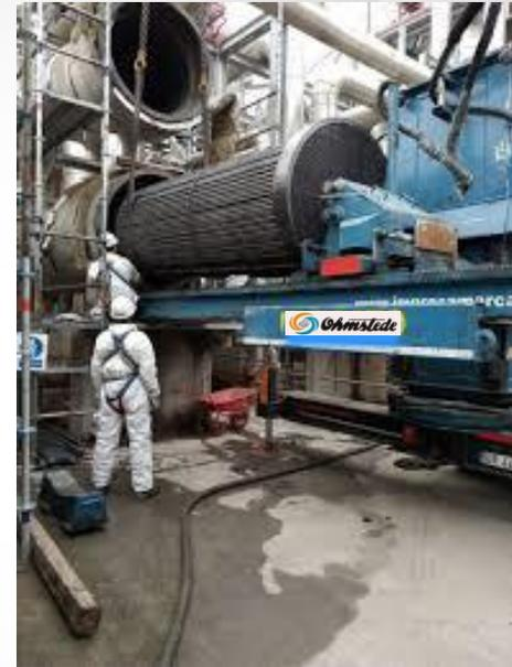
Breech-Lock exchangers are very unique and require specially trained / experienced personnel to effectively disassemble, maintenance and reassemble with leak free results.
